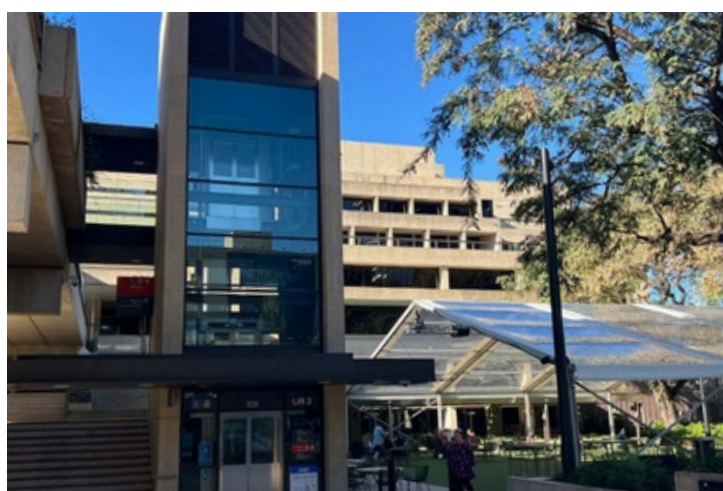
Cultural Centre Station busway, Melbourne St lift.
