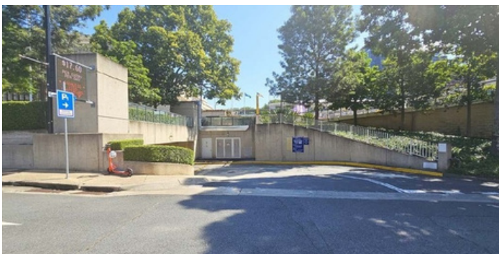
Performing Arts Carpark (P1), entry via Stanley St.
