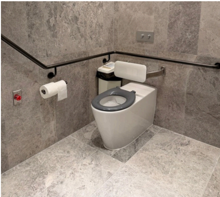
Accessible bathroom facility
